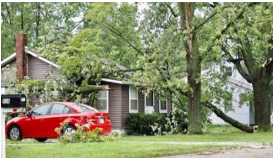
Figure 37 Damage from a Windstorm
