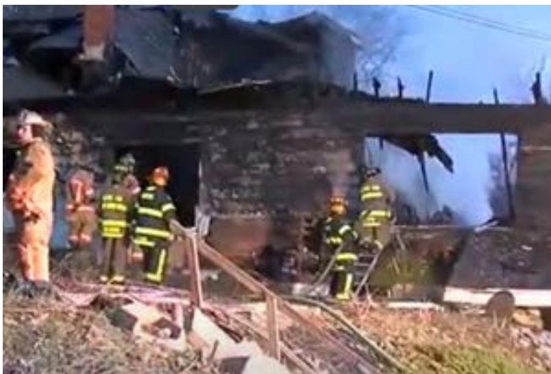
Figure 30 House Fire, near Aurora, IN
