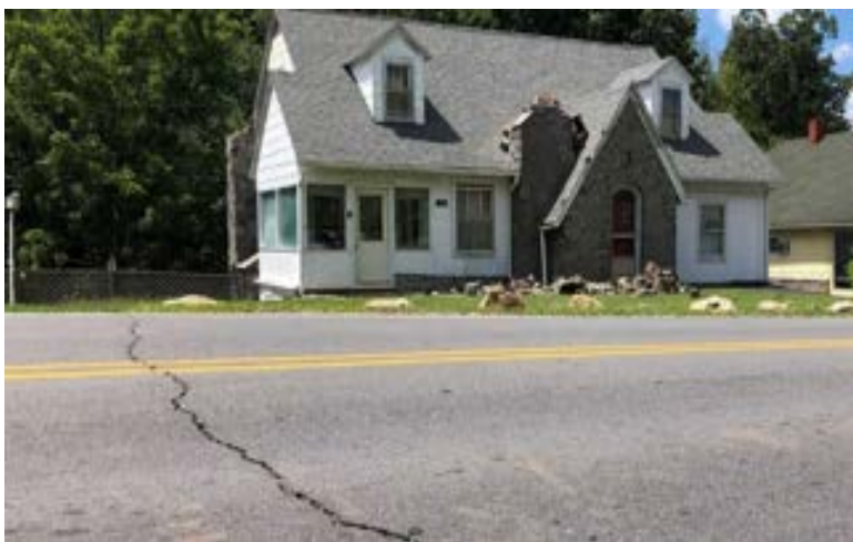
Figure 21 Minor Earthquake Damage
