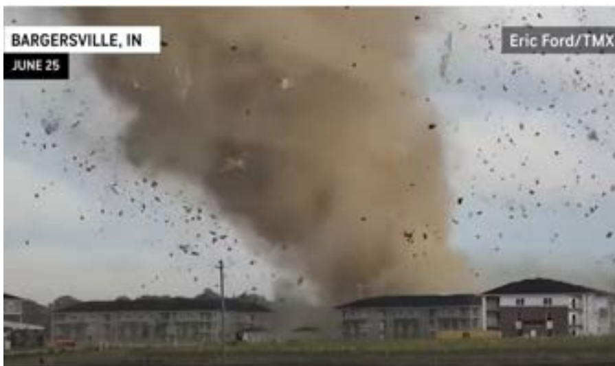
Figure 40 Debris Flying as Tornado Destroys Apartments under Construction
